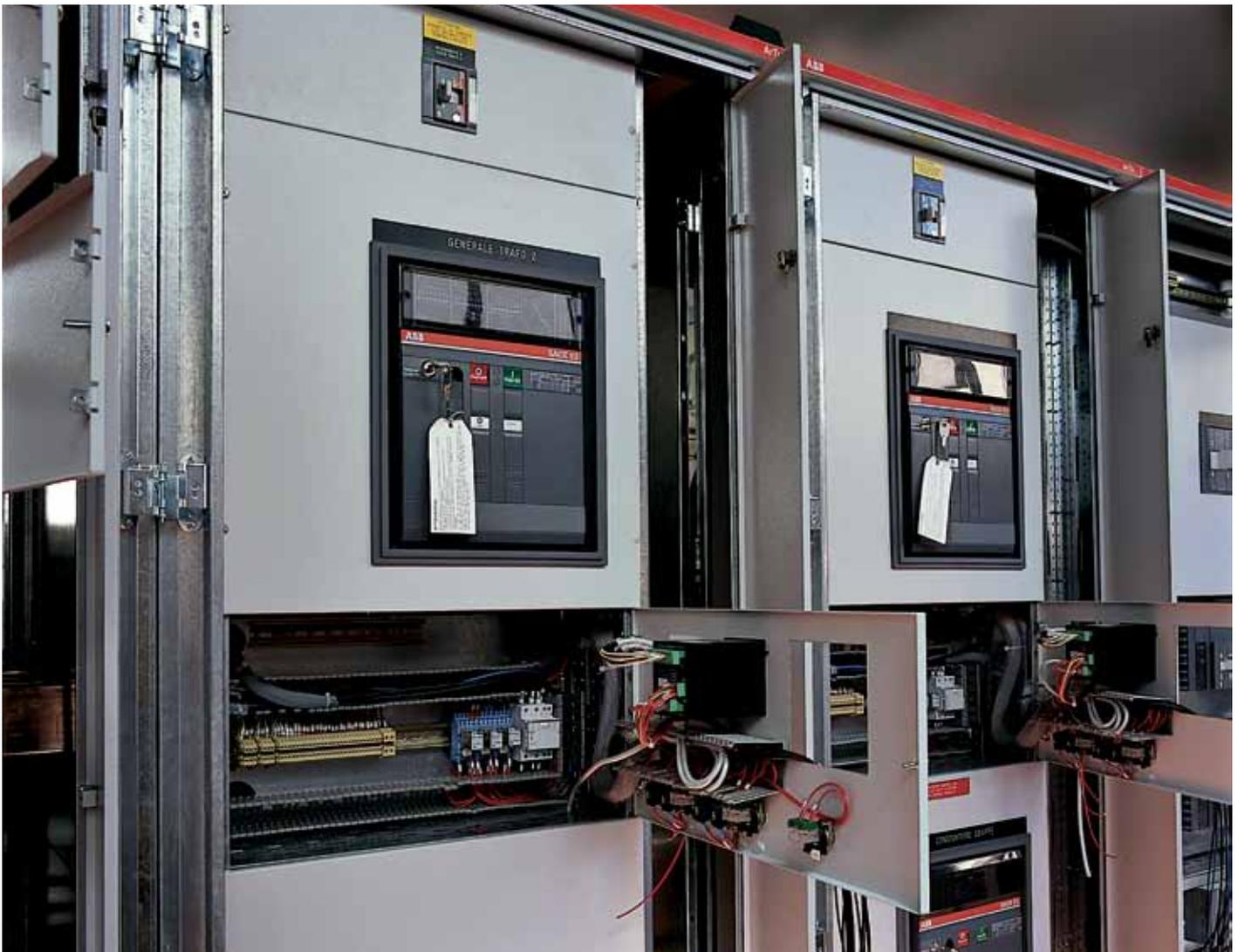
Within the K series of ArTu switchgear with 500, 700 and 900mm depths, segregation compartments of Form 2, 3 and 4 can be made in conformity with the IEC 60439-1 Standard.
