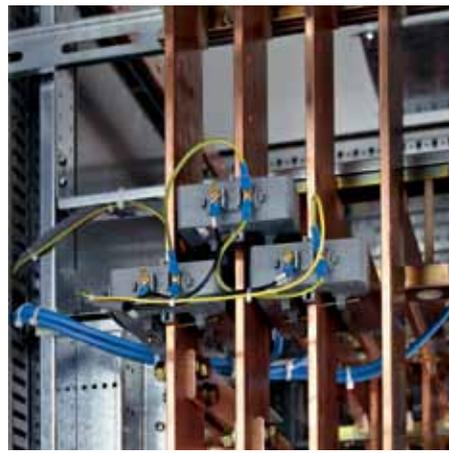
The extremely compact dimensions of the system allow the busbars to be mounted directly inside the switchgear, positioning them horizontally or vertically, on the back or on the side of the structure.
